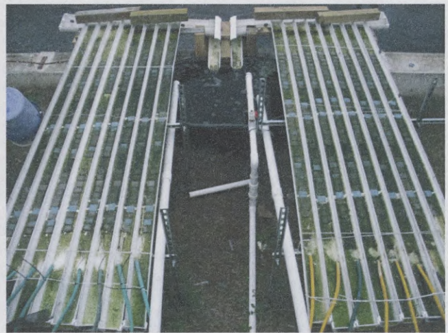
Figure 1. The algal turf scrubbing (ATS™) recirculating system at the Columbus Waterworks Inc. (South Facility).
